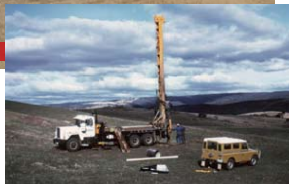
Langloh being drilled in the early 1980's.
